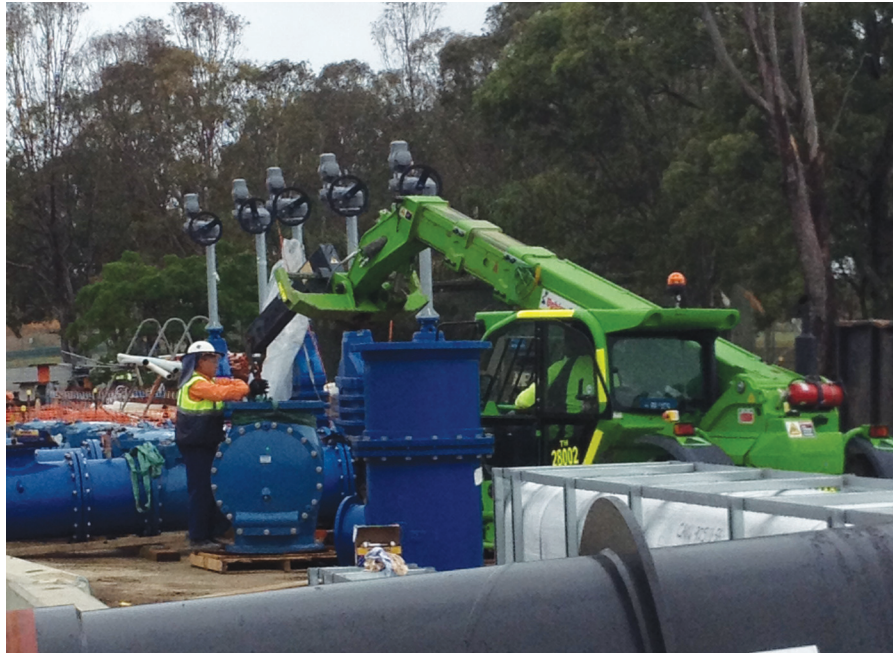
A telehandler at work on site
